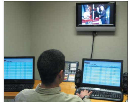
Digital Broadcast Customer Service Engineer Mike Regina prepares for operational training on a MediaFire system following installation.
